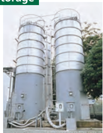
Material Storage SILO
