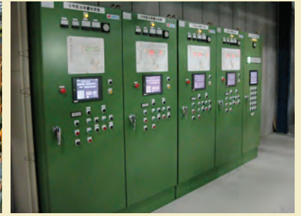
Powder and granule mixing system panel
