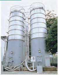
Material Storage SILO
