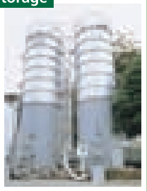
Material Storage SILO
