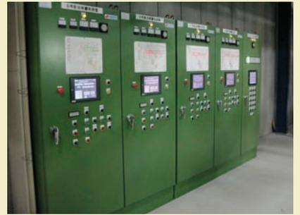
Powder and granule mixing system panel
